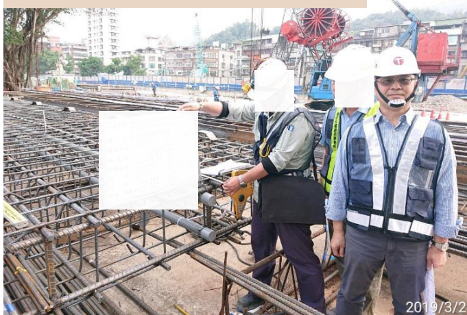
鋼筋籠查驗-基樁
