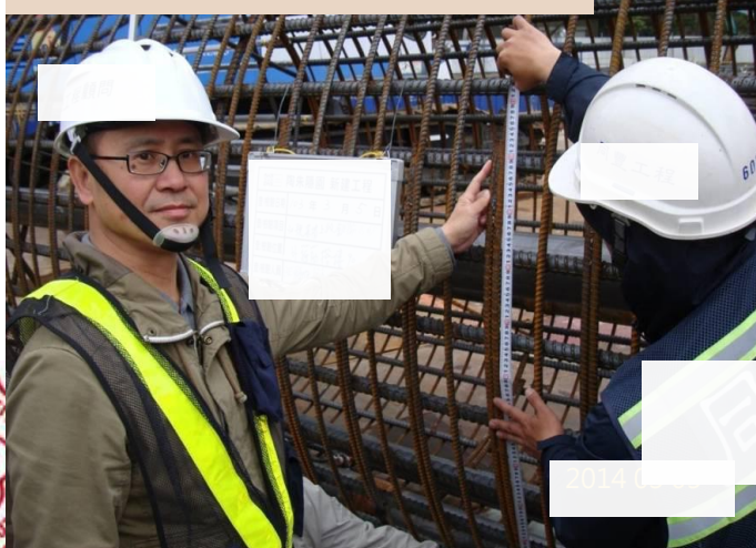
鋼筋籠查驗-基樁
